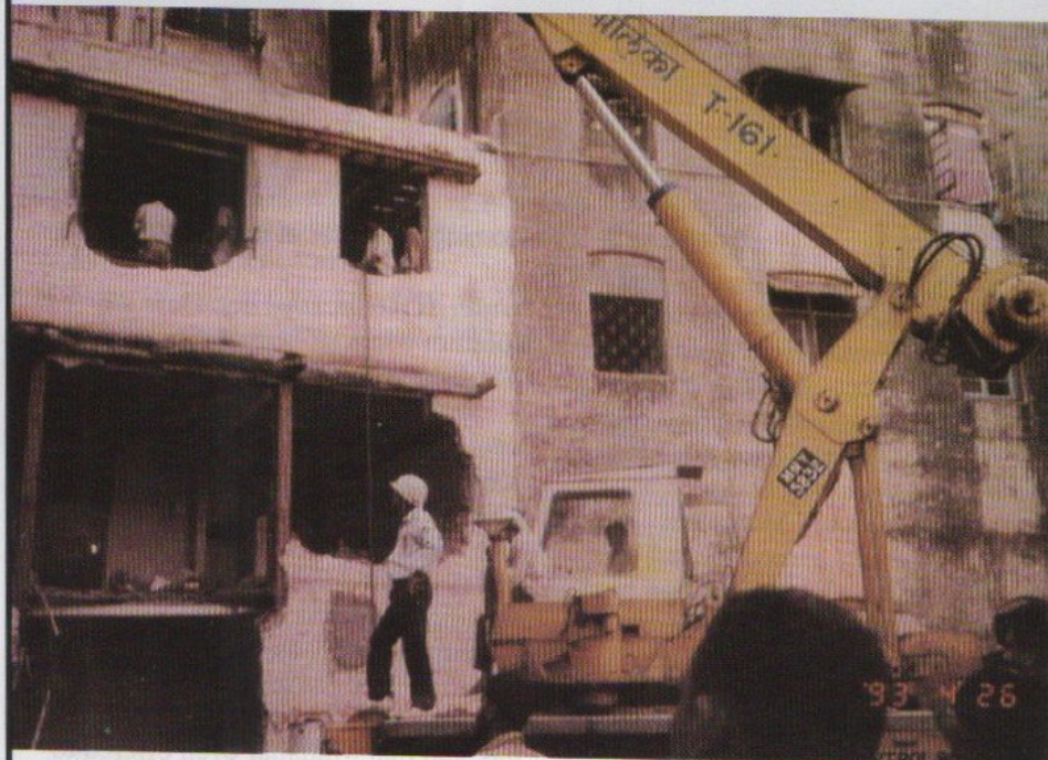
A demolition drive
