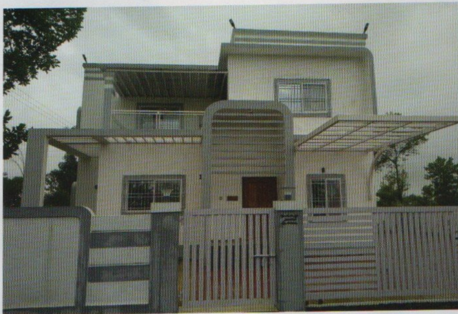
GenNext Villas - already handed over
