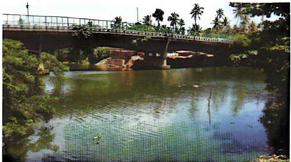
Karamana river and bridge - view from river bank at Thiruvallam
