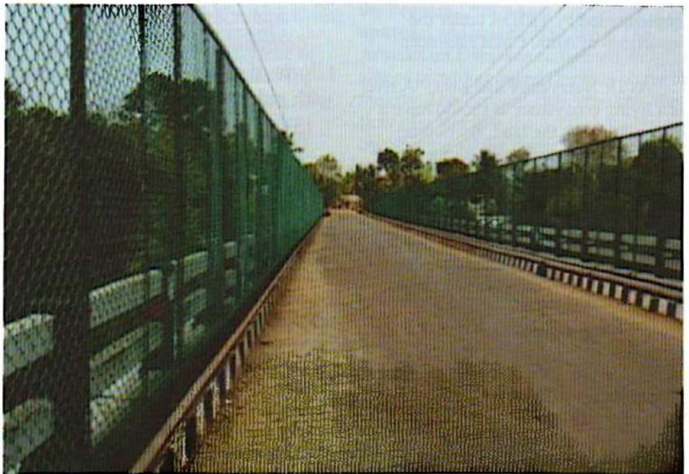
Chain linked fencing on the bridge across the river
