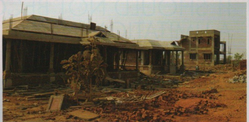
Construction work in progress of Nadumuttam villas at Banjara Hills.
