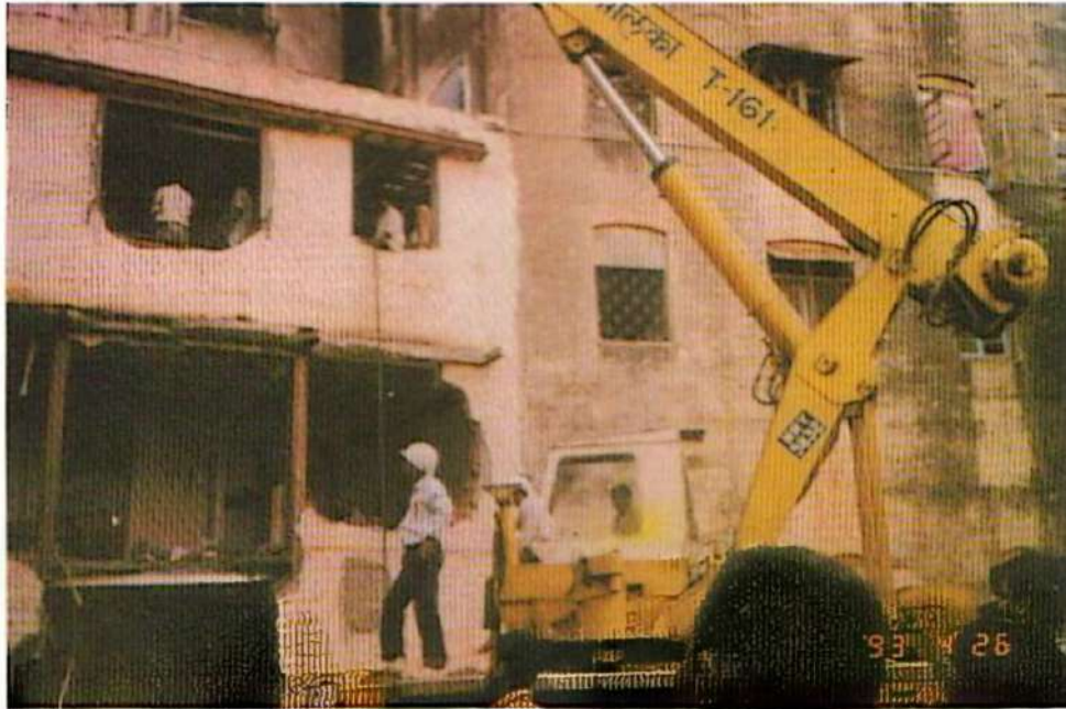
Demolition in progress
