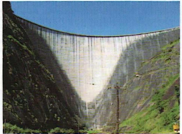
Idukki Arch Dam
