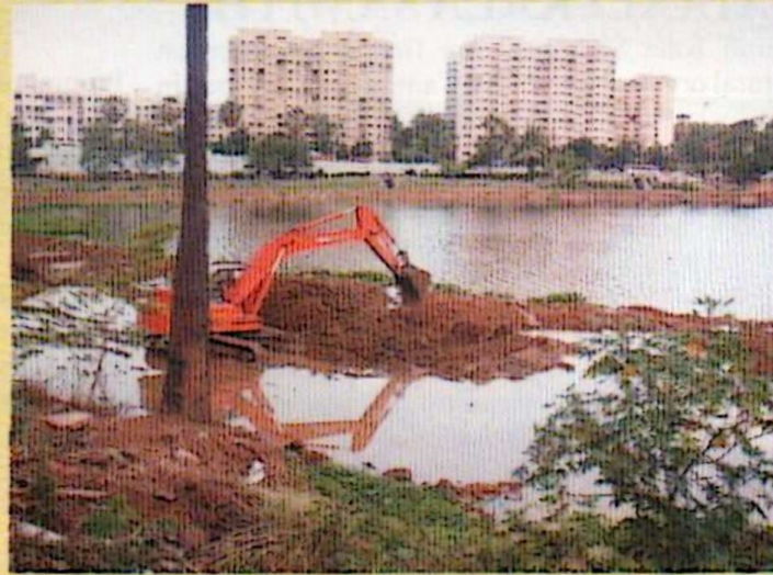
Desilting work at Powai Lake
