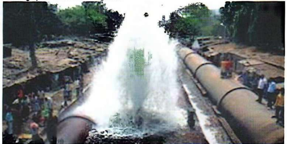
Ruptured pipelines wasting water in Mumbai
