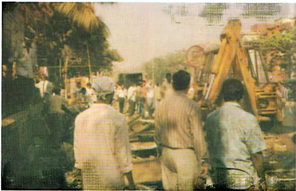
Demolition in progress
